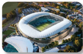
Sydney Football Stadium Redevelopment
