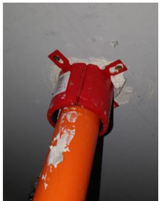
FyreCHOKE collar installed with conduit
