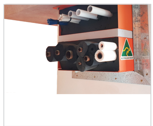
Double vertical FyreBOX installed above a doorway to allow for the provision of large amounts of services in a small space.
