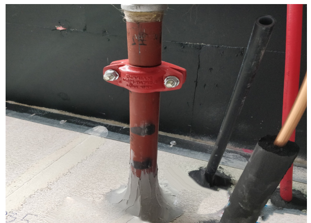
Traditional fire sealant penetration systems need the fire walls to be installed first, requiring extra couplings for pipes (above). Fire cables (below) cause defects when run through deflection heads.
