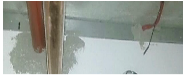
Traditional fire sealant penetration systems need the fire walls to be installed first, requiring extra couplings for pipes (above). Fire cables (below) cause defects when run through deflection heads.
