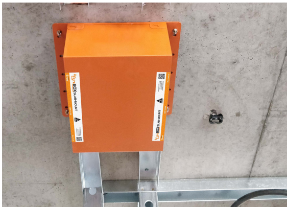
FyreBOX top plate, body and approved services all installed as standard to the soffit, with foam end plugs installed around the services.
