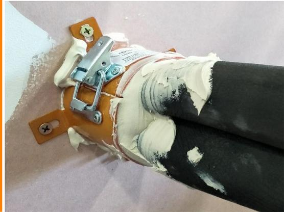
Where annular gaps exist between the services and the collar, back-fill these FyreFLEX® Sealant to the full depth of the collar.
