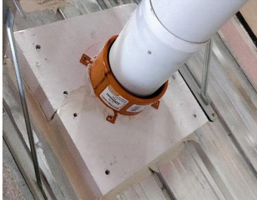
Speedpanel walls require a 60mm thick piece of FyreBOARD Maxilite® to be screw fixed onto one side of the penetration, before attaching the collar. See table below for screw fixings. Seal all gaps and perimeter with FyreFLEX® Sealant.
