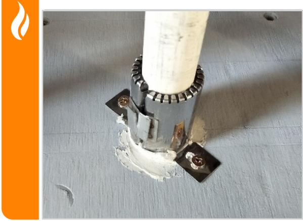
For the FyreCOLLAR Conduit, separate the two halves, fit them on either side of the service before sliding the halves back together.
