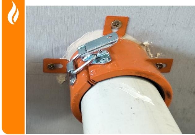
Use appropriate fixings as per page 13 to secure the collar to the wall/floor using all of the available the fixing tabs.
