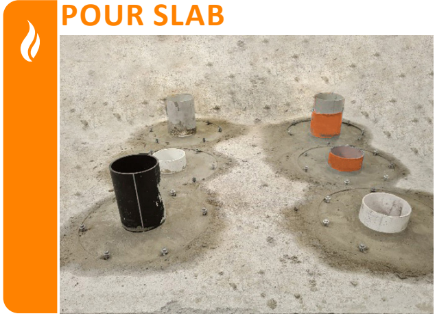
Pour the concrete slab, ensuring the collars remain firmly in place.
