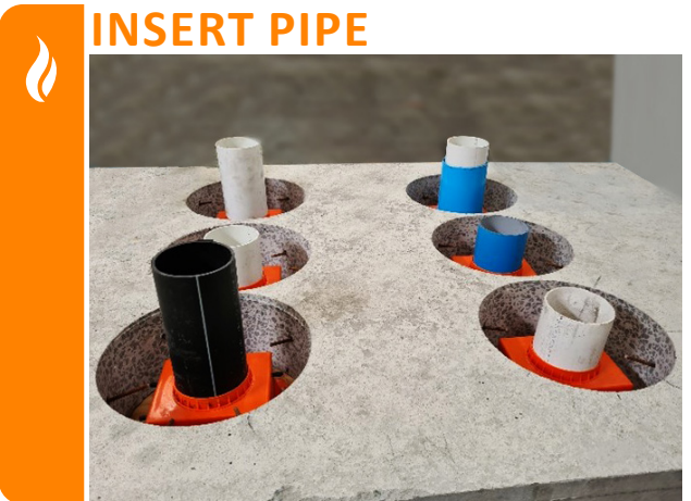
To ensure concrete does not fill into the collars, install a pipe former to the collar.
