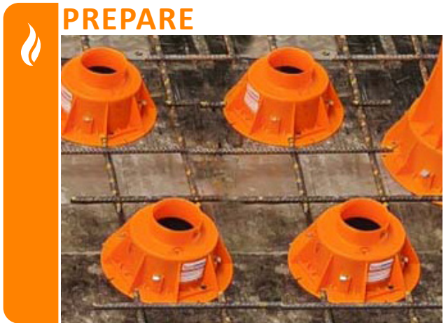
Fix the collar in place to the form work ensuring 50mm separation from edge to edge between each collar.
