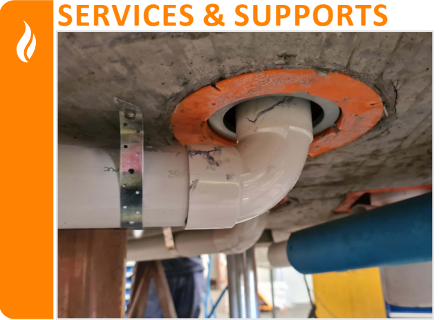
Once the slab is cured, connect the pipe/service, ensuring it is approved for the required FRL, as listed in this manual. Support as appropriate.
