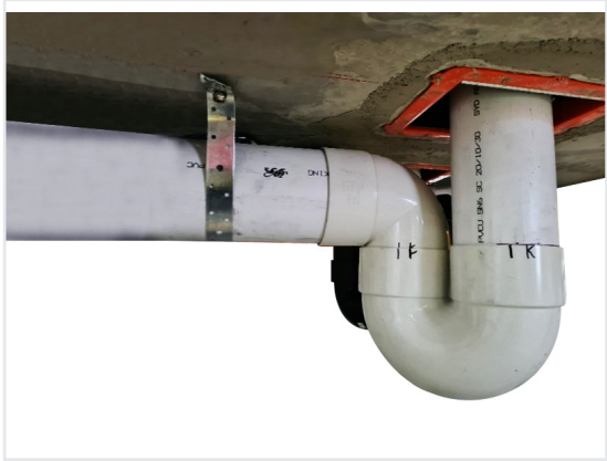
Once the slab is cured, the pipe formers can be gently tapped downwards to allow for connection of the pipe/service, ensuring it is approved for the required FRL, as listed in this manual.
