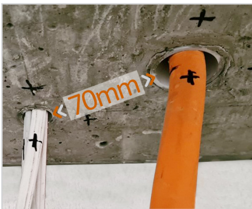
When setting the services in place, ensure that each is 70mm apart from the next (edge to edge).
