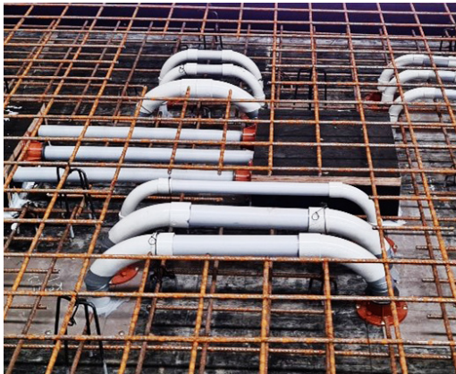
Set conduits in place in the concrete slab.
