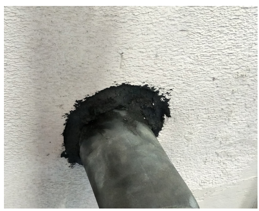
FyrePEX™ HP Sealant applied to a depth of at least 26mm from each side of the wall.
