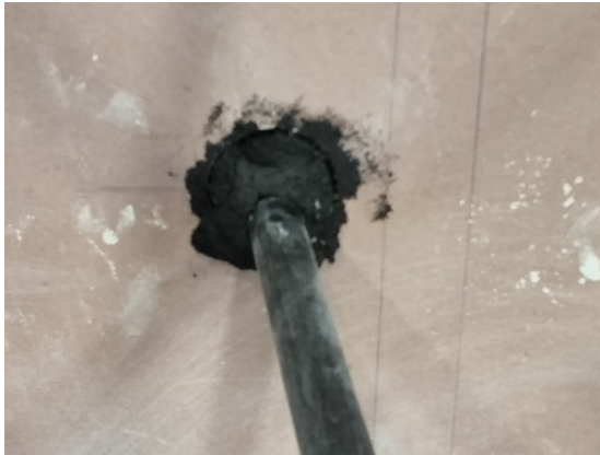
FyrePEX™ HP Sealant applied to full depth of plasterboard.
