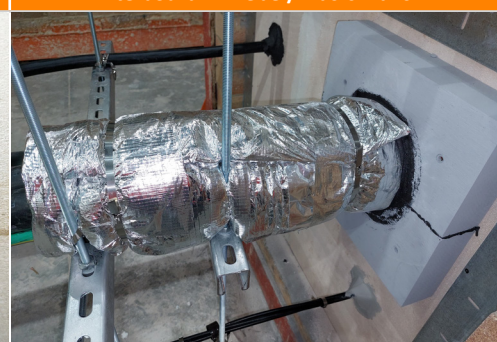
3. Large cable penetration thickened with Maxi-lite board in Hebel/Wasc walls
