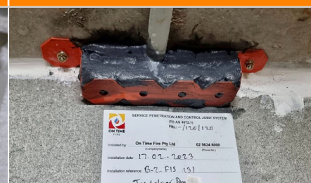
FyreSTRAP head of wall penetration
