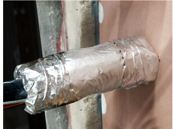
TWRAP TM secured on each side of penetration using three strips of reinforced aluminium tape applied around the wrap's circumference. TWRAP TM applied on both sides of the wall. Alternatively, apply steel ties 50mm from each end and at 150mm centres in between.
