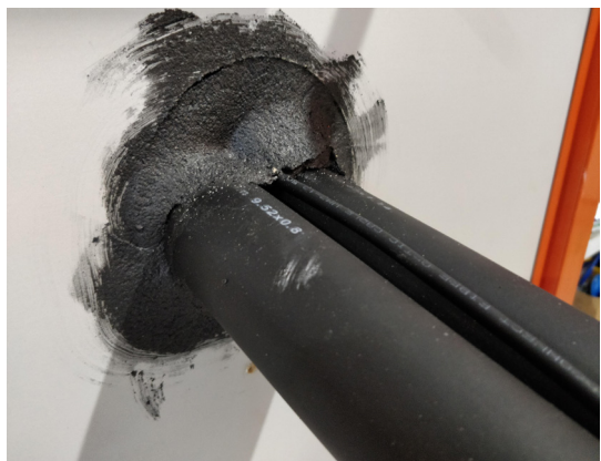
FyrePEX™ HP Sealant applied to full depth of plasterboard.
