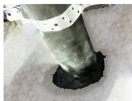
FyrePEX™ HP Sealant applied to depth of at least 60mm from top side of floor slab.
