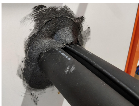
FyrePEX™ HP Sealant filled to the full depth of the plasterboard on both sides of the wall.
