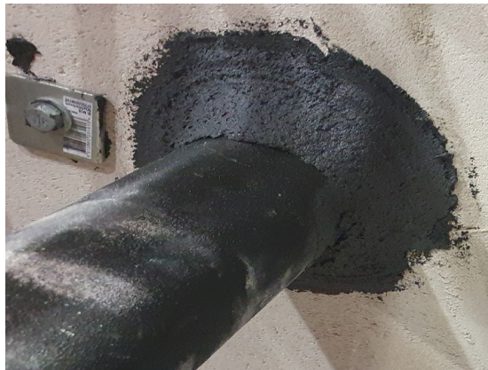
FyrePEX™ HP Sealant applied to depth of at least 60mm from one side of the wall with fillets if required.
