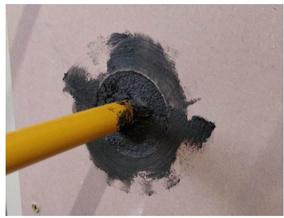
FyrePEX™ HP Sealant filled to the full depth of the plasterboard on both sides of the wall.
